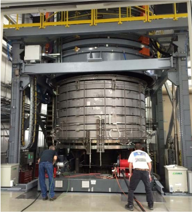
Figure 4. Technicians ensure proper placement before lowering heat treat furnace
