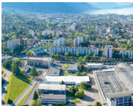
Pfeiffer Vacuum Technology AG announced in May 2023 a seven-year, €75 million investment plan for its Annecy site. (Source: heat processing)
