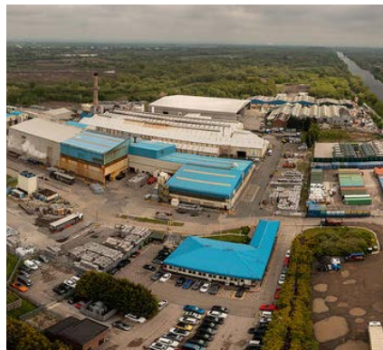
With the recently awarded grant by the Department for Energy Security & Net Zero, Novelis' Latchford plant will test the use of hydrogen on one of its recycling furnaces in a demonstration phase in 2024. (Source: Furnaces International)
